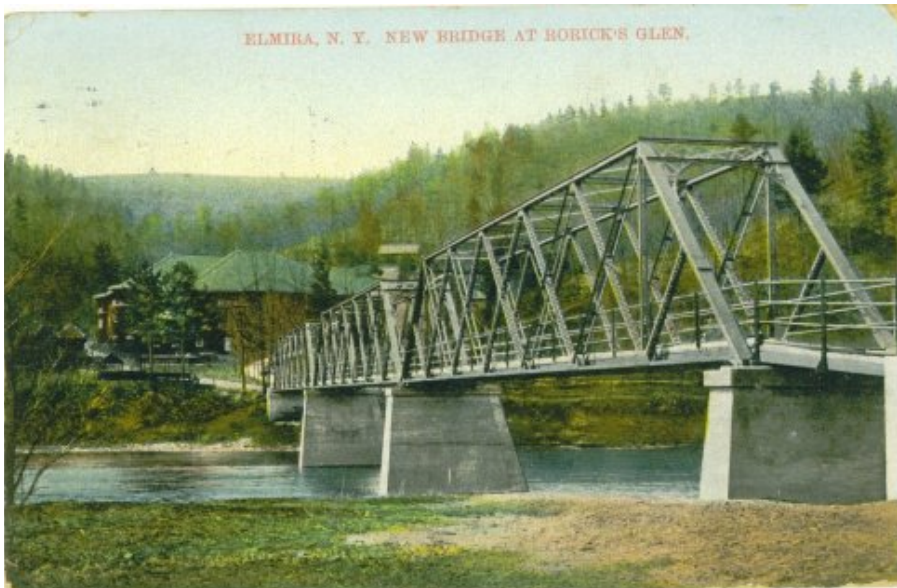
The new steel bridge at Rorick's Glen with the theater in the background
